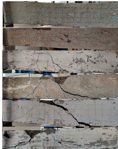
Figure 3 Crack patterns after testing (see online version for colours)
