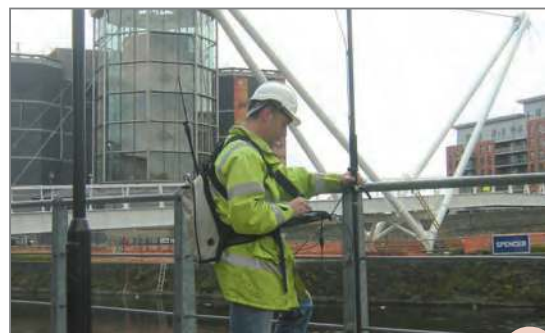
Figure 5.22 Surveying the footbridge
