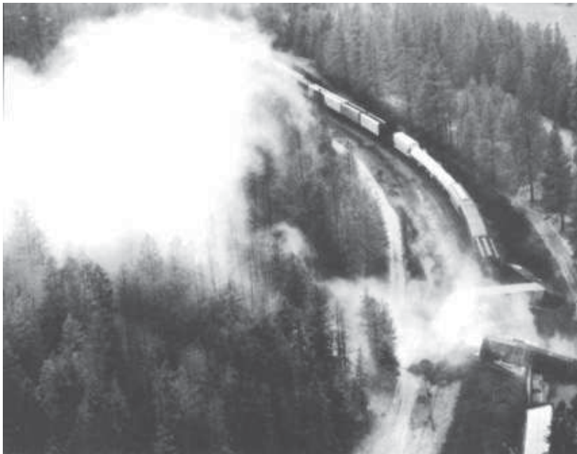
Figure 8.28 Low-altitude, oblique aerial photograph of chlorine spill resulting from train derailment near Alberton, MT. (Courtesy RMP Systems.)
