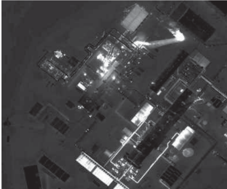
Figure 4.22 Thermal imagery from the TABI-1800 system, acquired over a natural gas processing facility and power plant near Balzac, Alberta, Canada. Light tones indicate higher radiant temperatures. (Courtesy ITRES, Inc.)
