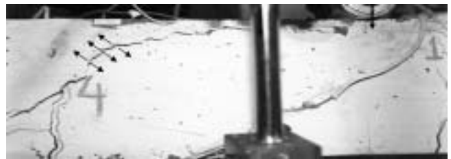
Fig. 8—Shear crack meeting vertical flexural crack below load at failure in Specimen B0-900.
